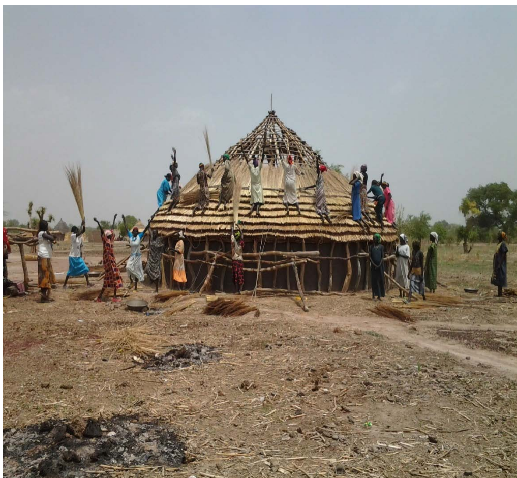
Figure 5: Caption of South Sudan women constructing a house and a good venue to reach women for TB education and screening
